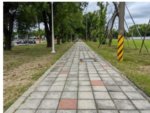
Permeable Pavement of Sidewalk
