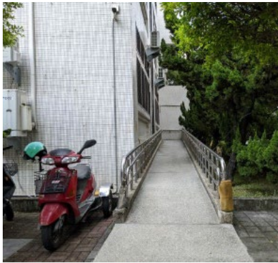
Barrier-free Ramp of Administration Building
