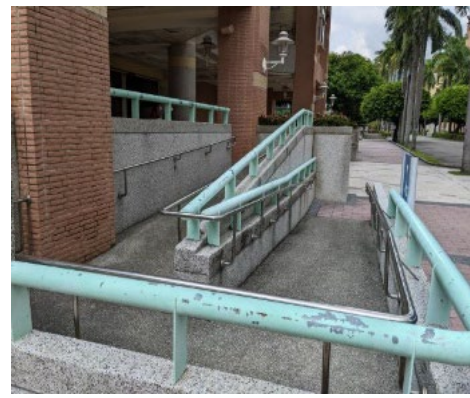
Barrier-free Ramp of Engineering Hall
