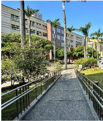
Barrier-free Ramp of Innovation and Research Building
