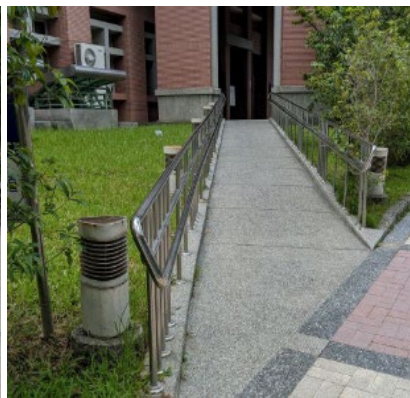
Barrier-free Ramp of Management Hall
