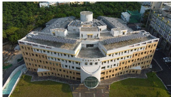
The solar power generation system on the top floors of the Machine Tool Building
