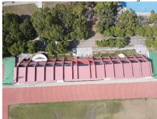
The solar power generation system on the Motorcycle Parking Lot (3)
