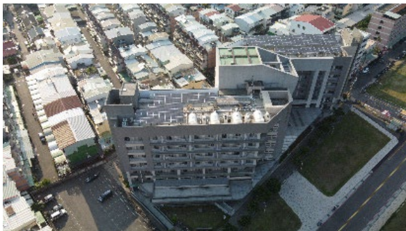
The solar power generation system on the top floors of the Chin-Yi Dormitory
