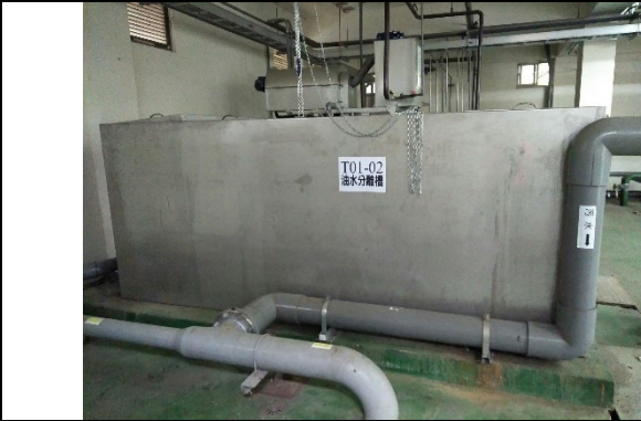
Original sewage well
