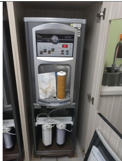
Replace the water dispenser filter
